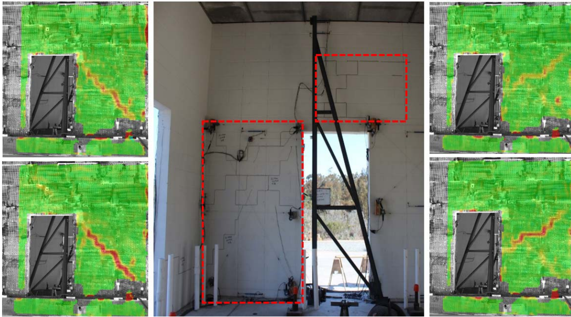
Figure 14: Post mortem crack pattern observation on wall 1 and comparison with characteristic full field images
